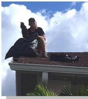
Michelle Collins, on the roof, cleaning the gutters of Faith Church!
